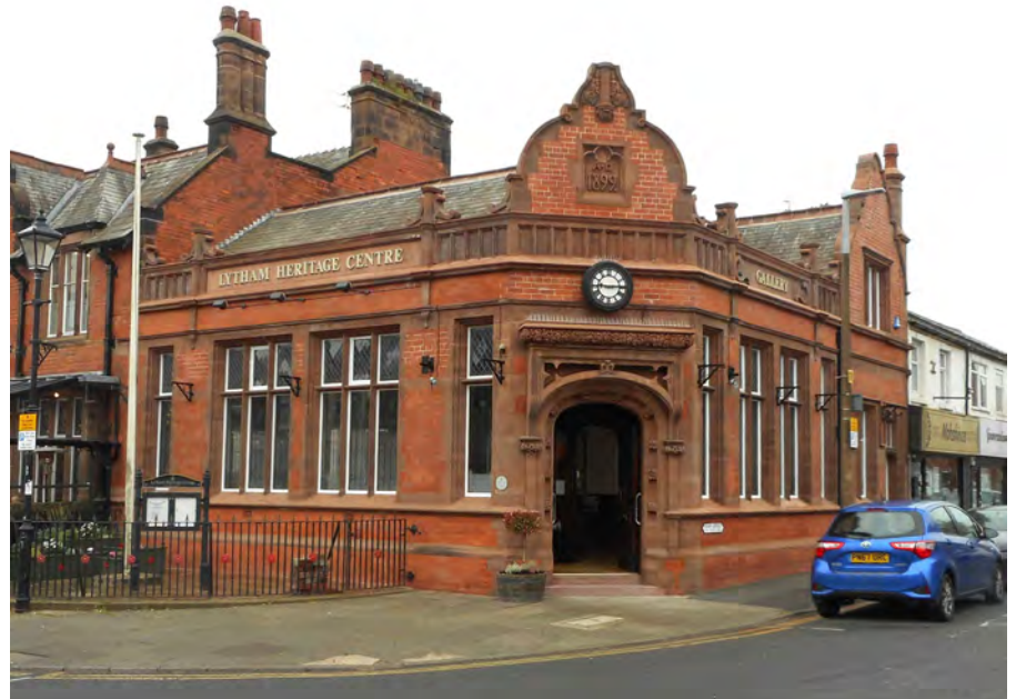
The scaffolding removed to reveal the superb looking refurbished grade II Lytham Heritage Centre (photo David Forshaw)
