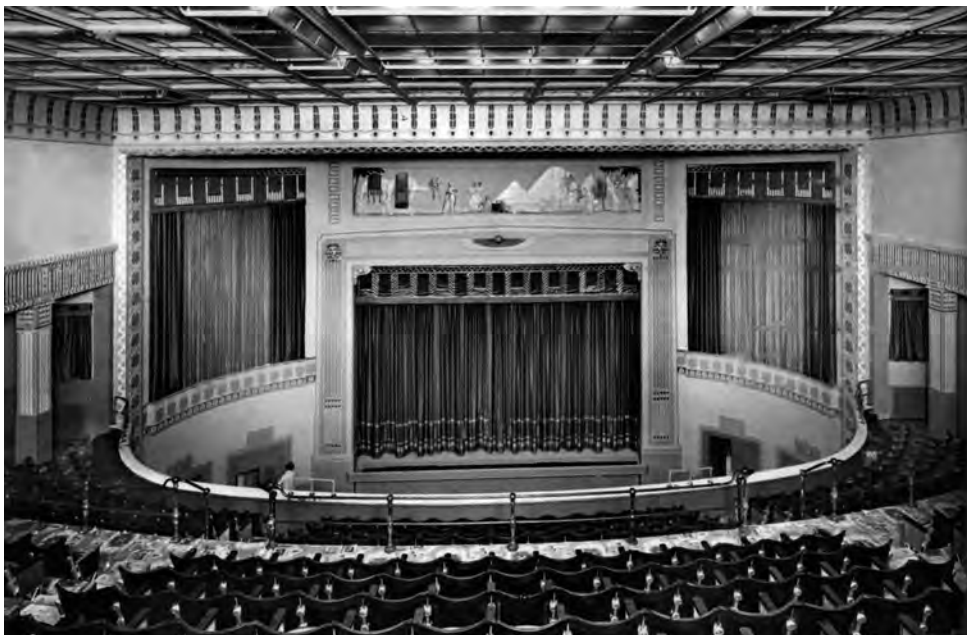
Interior view of the Palace Cinema, Clifton Street, Lytham, 1930 (Lytham Heritage Group Archives)
